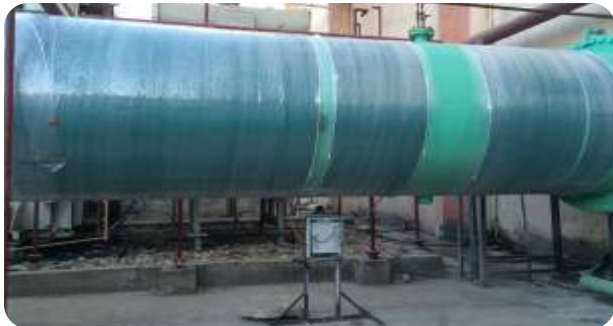
Pipe Diameter: 1.6 mtr. (63 inch) • Waterflow: 15,000 m³/hr
